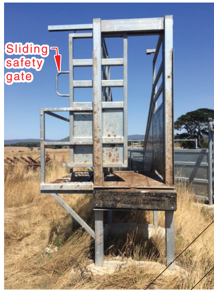
Figure B.3(K) — Sliding safety gate at front of ramp to allow safe access to close/open livestock crate door
