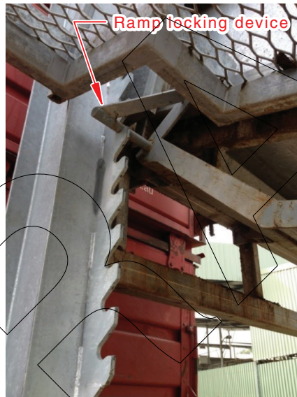
Figure B.3(P) — Ramp locking device
