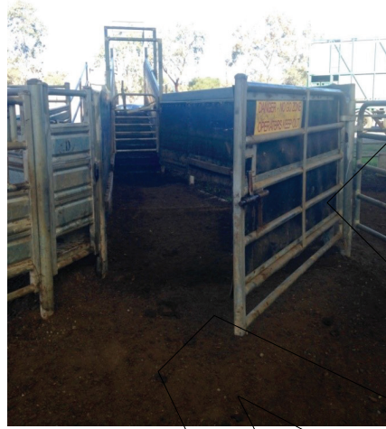
Figure B.3(T) — Forcing pen with no blind corners and with infill sheeting
