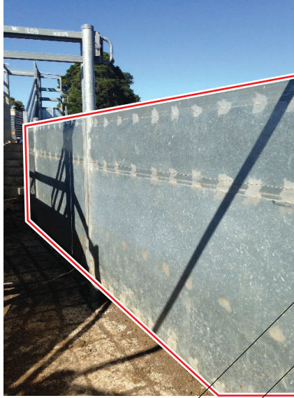
Figure B.3(N) — Infill on walls of ramps
