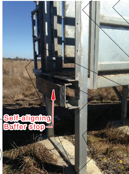
Figure B.3(H) — Self-aligning buffer stop on front of ramp
