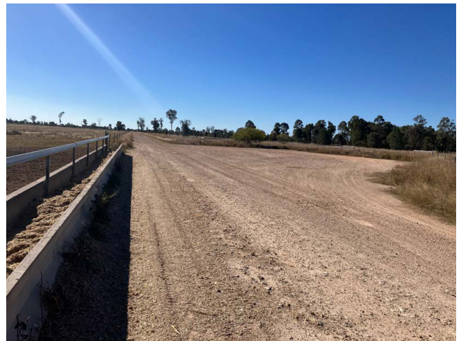
Figure 6: Shared stock lanes and roads designed to allow for feed truck turn around at each bunk. Left: dual feed road servicing bunks on both sides. Right: feed road with one bunk and turnaround at the end of the bunk.
