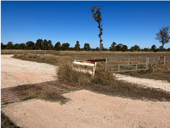
Figure 5: Gate and grid to assist in controlling stock movements without impacting feed trucks
