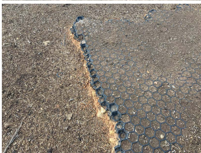
Figure 7: Examples of pad reinforcement. Left: Concrete apron and extended gravel pad. Right: plastic grid mesh reinforcement.
