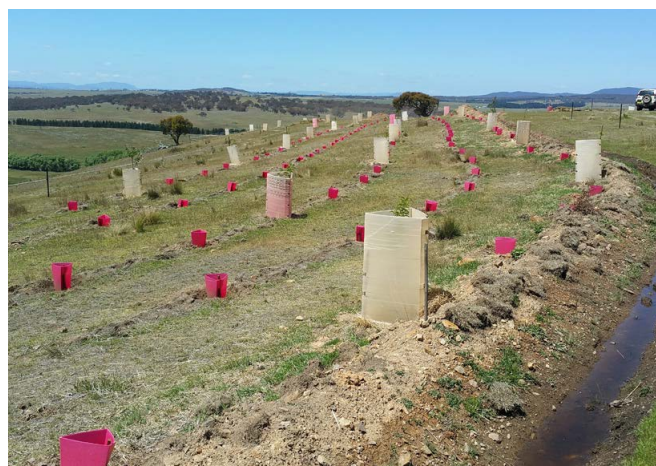
Figure 8: On-contour swale with downslope vegetation Source: Mulloon Institute
