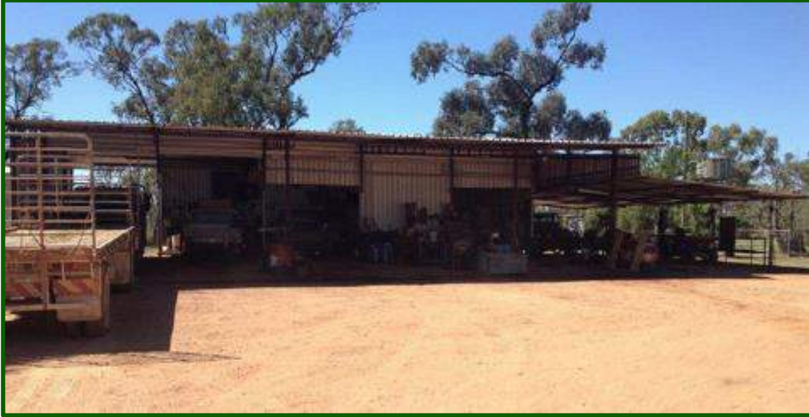
Craiglee Workshop of 130sq m, with concrete floor, steel posts and galvanised roof.
