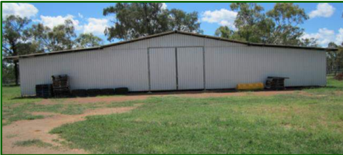
Craiglee Truck/Hay shed of 336sq m, earth floor, and metal roof.
