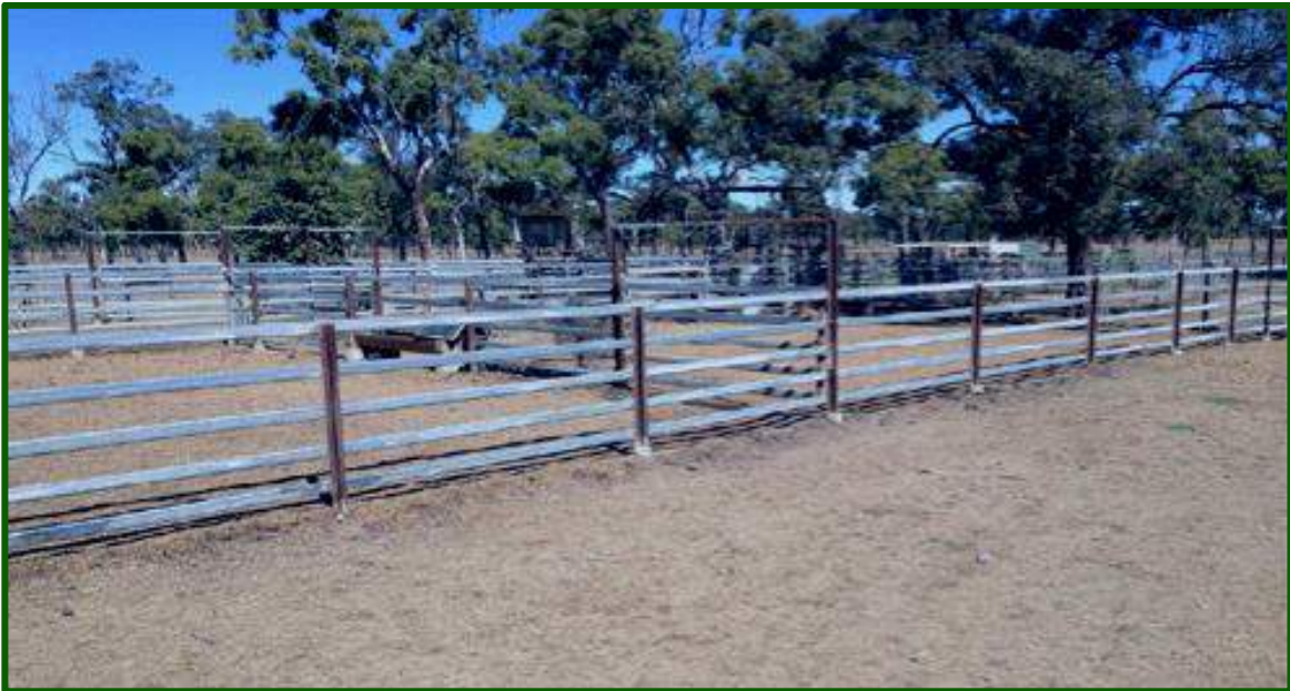
Yards comprising railway line posts, 5 rail galvanised cattle rail, and cable, and some portable panels. Some gates have slam shut latches.
